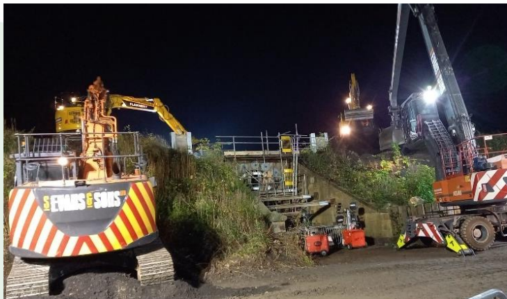
Underpass works being completed between Seaton Delaval and Newsham.
