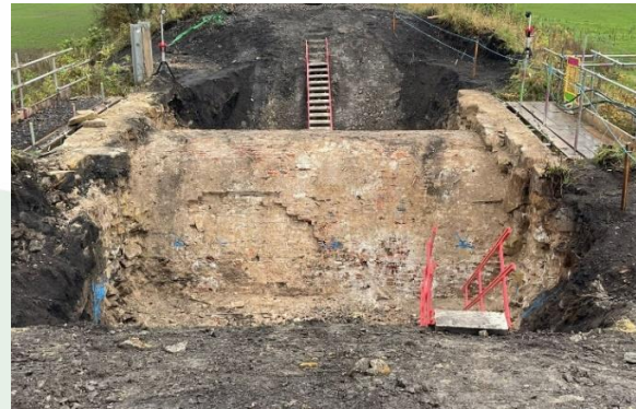
The top of arch after the tracks were removed.
