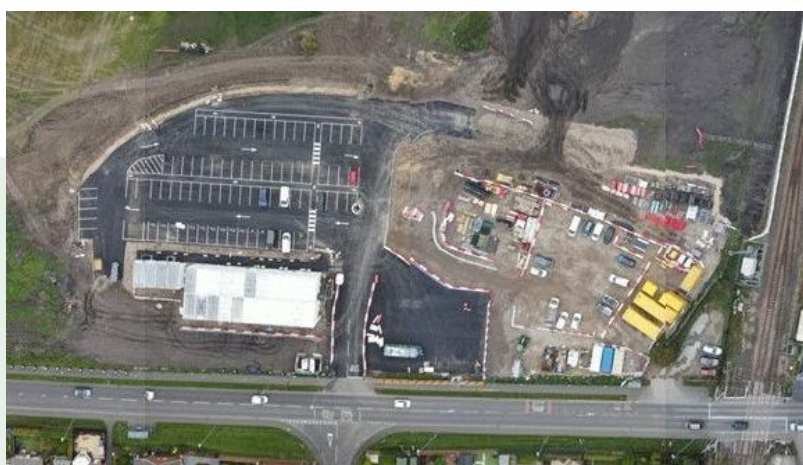
Aerial view of the works taking place at Newsham station
