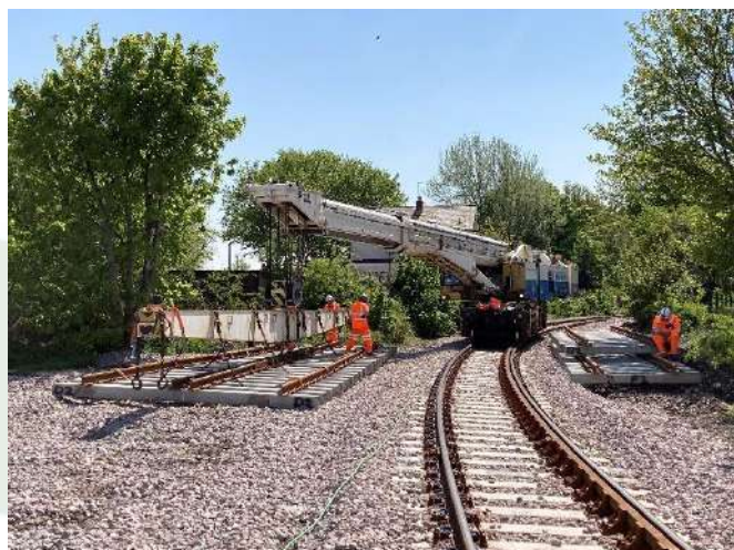
Installation of new track crossing panel at Redhouse Junction
